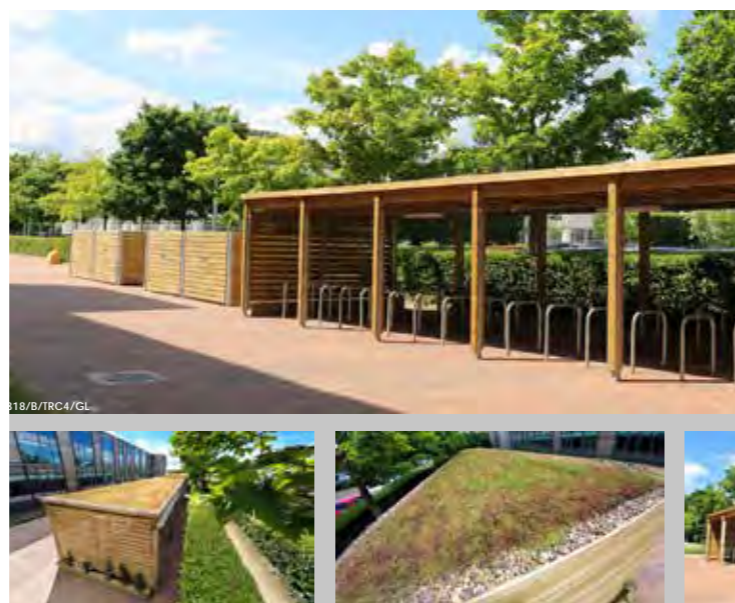
Figure 2 Furniture Type 5: Bicycle Shed with Sedum roof Supplier: Langley or Similar Approved Size: Varies Material: Steel and Timber
