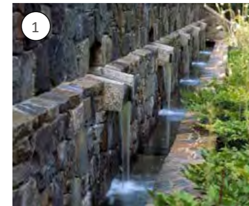
Water spouts protruding from haha
