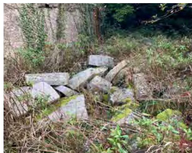
Concrete Block Wall
