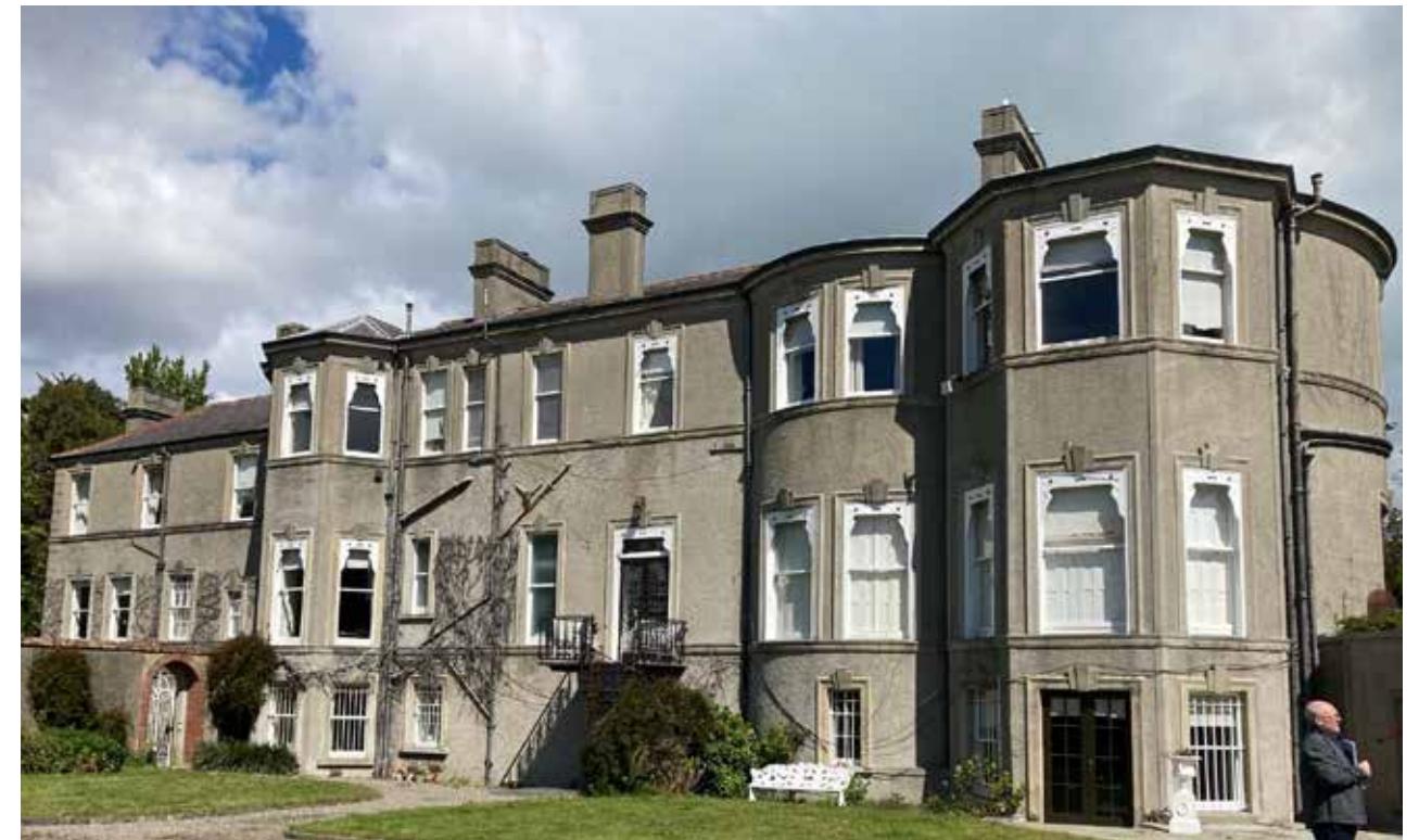
Dalguise House - Existing
