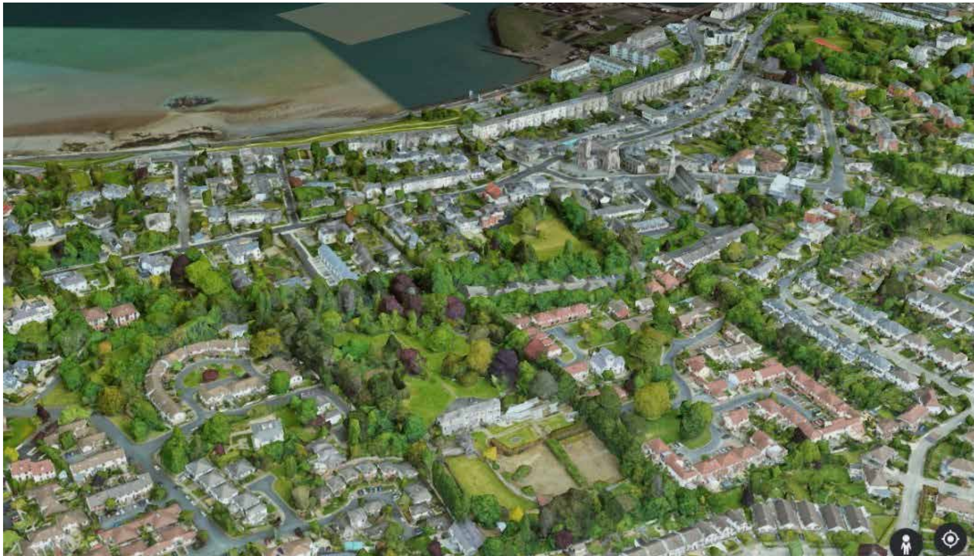
Figure 1 - Site aerial view
